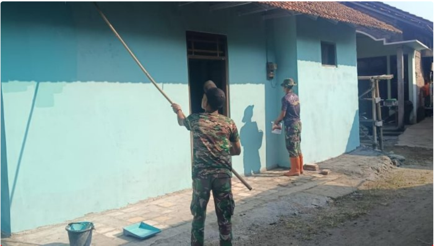
(Foto istimewa) Pengecatan RTLH TMMD 116 Kodim 0722/Kudus
